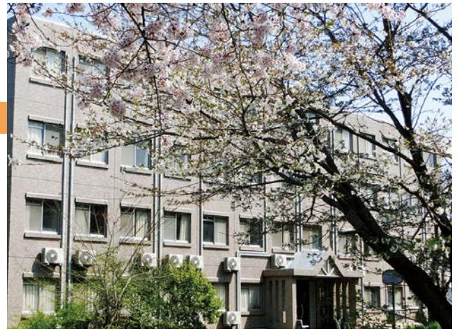
▲学寮風景 Hall 5 is placed on the eastern side of the premises.
