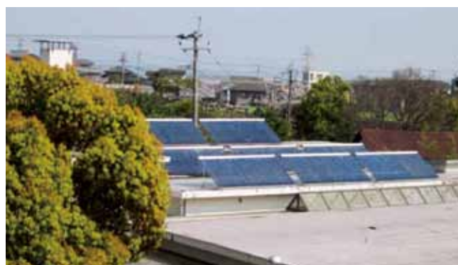
▲ Akeno-ryo has installed a solar hot water supply system. Now, you can enjoy a warm, comfortable bath. We have cut fuel cost and reduced CO2 emission as well.
